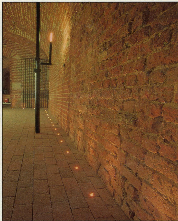
Fibre optic uplights recessed into the floor of the basement.
